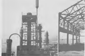
THE CHEMICAL combination or union of hydrogen and nitrogen to form ammonia takes place in the presence of an iron catalyst under high temperatures and pressures. The change occurs in an ammonia converter, above, which is sited in the ammonia synthesis section. Structural members of the Antilles' stand against the sky, center. Instrumental, electrical and machine work is done here. Construction work shapes the towers of the Aruba Chemical Industries plant, right, on the west side of the site.
